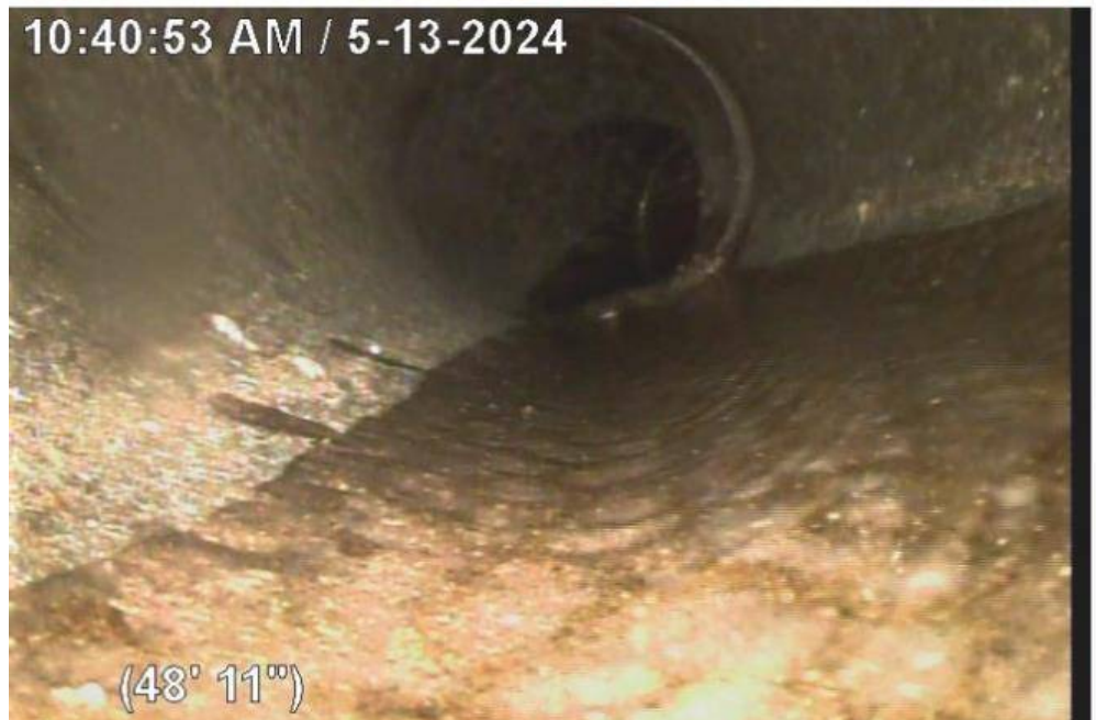
Examples of the serviceable portions of the Clay pipe beyond the damaged sections.
