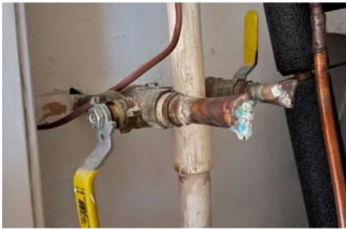
Pipes CUT / Valves CLOSED WRONG!
