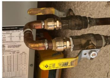
Pipes LOOPED / Valves OPEN RIGHT!
