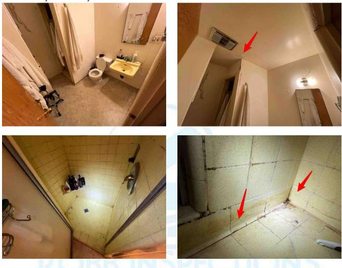
WALLS AND CEILING Needs Attention: There is moisture damage on the walls / ceilings.
