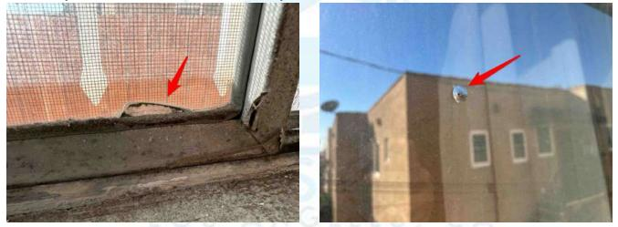
the windows do not work well and are generally difficult to operate. They will need adjustments or repairs to operate properly throughout the units.
