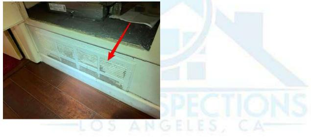
This air return is drawing it's "supply air" from the walls / ceilings in an unsealed return. This is no longer recommended as this can draw in odors, dust, etc from inside the walls / ceilings, and is less efficient as this air requires more heating / cooling, and causes the conditioned house air to be expelled through house cracks and gaps to make room for this new air to enter. It is recommended that a return duct and grill be fully sealed.
