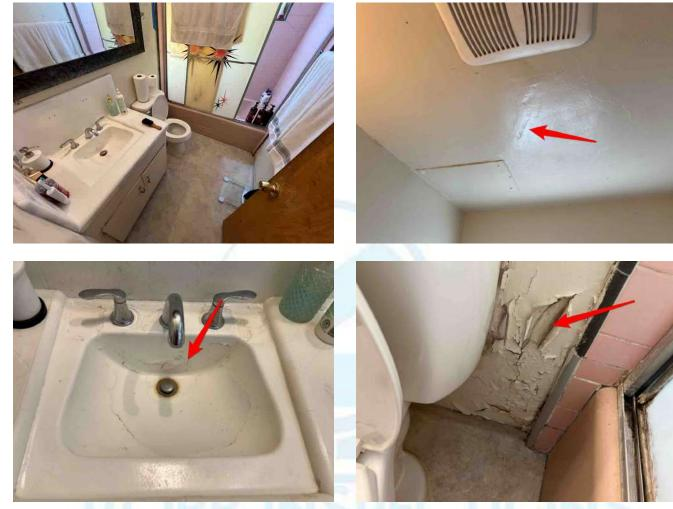
WALLS AND CEILING Needs Attention: There is moisture damage on the walls and ceilings.
