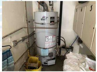
LOCATION CONDITION Needs Attention: There is no drain pan below the water heater and this is advised in case the water heater leaks so that the water can be carried away from the living space.
