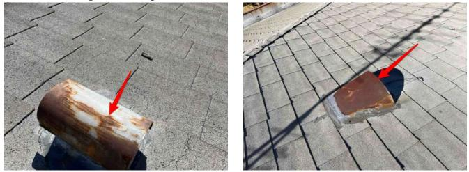
There are gaps in the mastic, where the mastic is cracked and in need of repairs.
