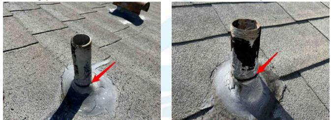
The flashings have been covered over with mastic which is a temporary solution and will require regular maintenance to help ensure a leak free condition.
