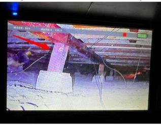
The piers and posts that hold up the structure are undermined in areas where the earth under them has been removed. They do not have full bearing on the soil and cannot give full support.
