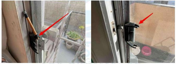
the sliding glass doors do not appear to have tempered glass or a safety film installed on them. Having one or the other reduces the danger of bodily harm should the glass be broken and in some cities is required at the time of sale.
