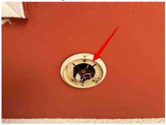
The unit 4 smoke alarms appear old, the manufacturer recommends that they be replaced after 10 years to ensure safe operation and reliability.
