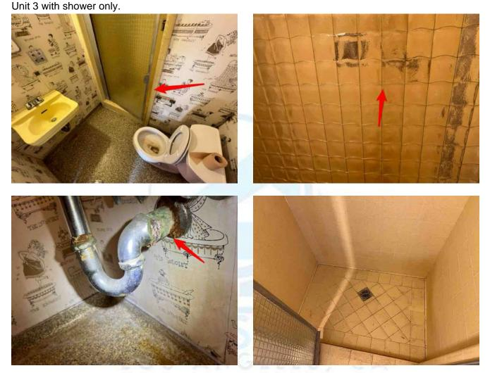
DRAIN Not Acceptable: The drain has some corrosion / rust in areas.
