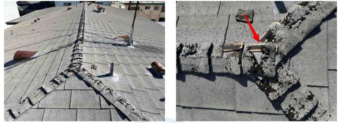
There are areas of damaged and deteriorated shingles.
