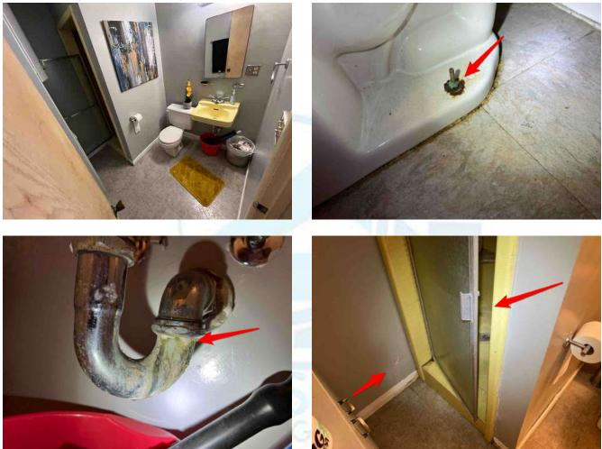
WALLS AND CEILING Not Acceptable: There is moisture damage on the wall outside the shower
