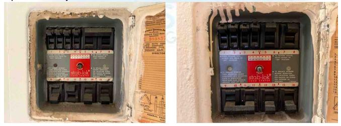
The circuit breakers in the panel(s) do not have a complete directory so it is not known what each breaker controls (or protects) in the building.
