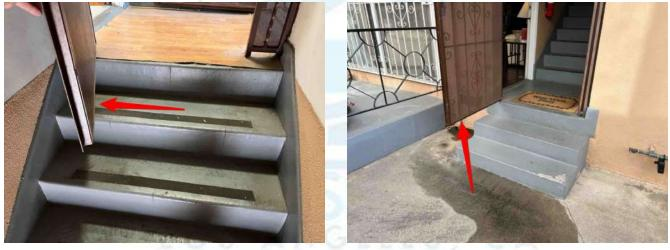
there are interior doors that have some damage at the base, missing or no door stops and that are out of adjustment and could use repair throughout the units.
