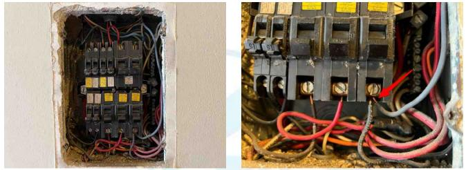
This panel and circuit breaker system is an old "Stab-Lok" or "FPE" (Federal Pacific Electric) system. It is past the end of its expected life span. As with all older systems it will be more prone to failure due to its age and design. Some of these older systems have a reputation for unreliability, failing to trip, jamming, or overheating. Electricians may recommend the panel be replaced for safety.
