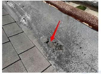
Note: There are areas where water will pond on the roof as is the nature of flat roofing, these areas will typically wear out quicker than the remainder of the roof.
