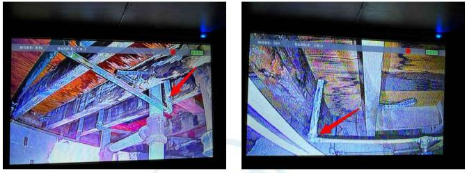
There are copper to galvanized steel piping connections without the proper fittings that keep these dissimilar metals apart (dielectric or brass fittings). These metals react against each other without these fittings and the galvanized piping corrodes faster. Even proper fittings are just a temporary solution and will not correct or stop corrosion or handle the problems of pipes rusting out. The remaining galvanized pipes will need to be replaced in time.
