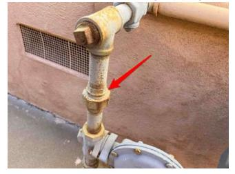
There are no or improper gas line sediment traps installed in areas such as at the heater and water heater as required by today's standards.
