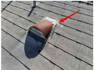
There are flashing with missing rain / weather caps.
