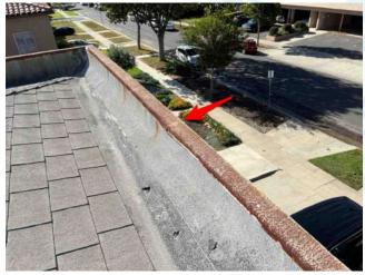
The metal flashings are rusting and corroded in areas.
