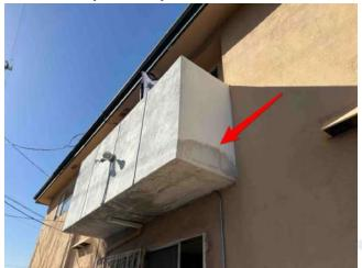
There are cracks in the surface of the balconies for units 3, 4 and 5, these should be repaired to prevent moisture intrusion into the structures.
