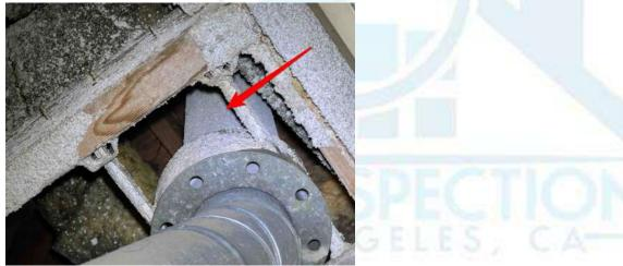
The roof weather / rain cap is missing and the vent / caps are rusted in areas.
