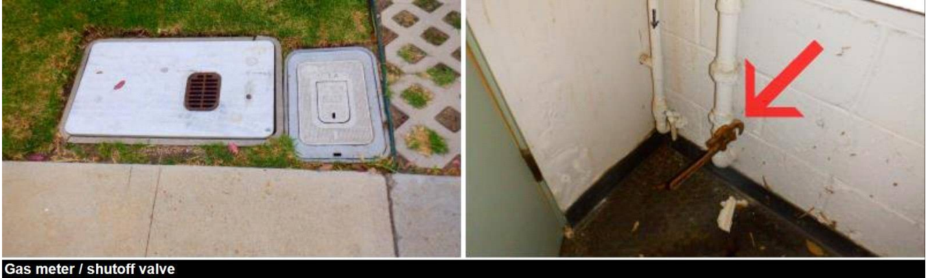
Gas meter / shutoff valve
