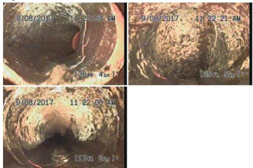
In the vitrified clay main sewer pipe, there are root intrusions at the joint areas. Root intrusions at the joint areas of a vitrified clay sewer pipe are common and can normally be maintained with regular sewer line cleanings. However, if these root intrusions are left un-maintained for extended periods, they can create blockages in the system and potentially damage the pipe itself.
